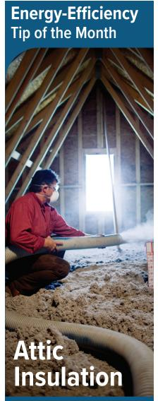
Even in summer months, adding insulation to your attic can keep your home more comfortable and save energy used by your cooling system. If your attic insulation is level with or below your floor joists (meaning you can easily see your joists), you should add more. If you can't see any of the floor joists because the insulation is well above them, you likely have enough insulation.
